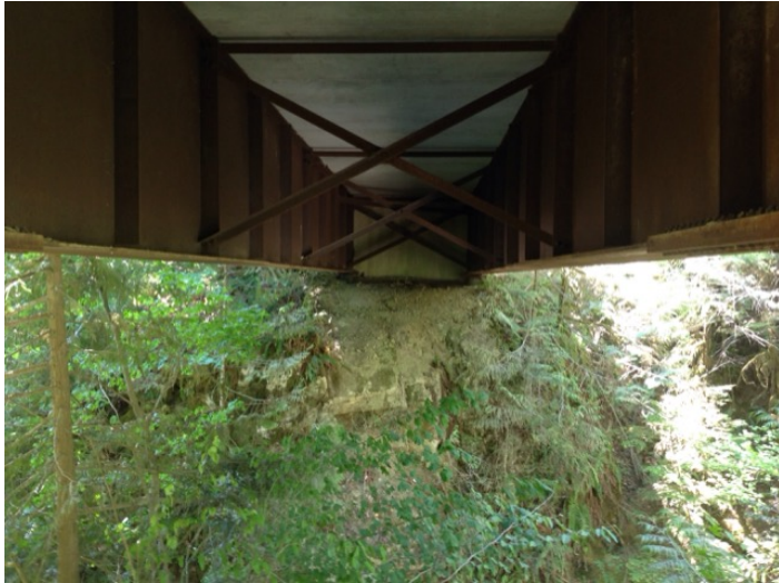
Right Bank Abutment when facing downstream
