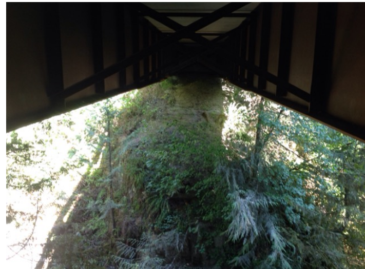
Left Bank Abutment when facing downstream
